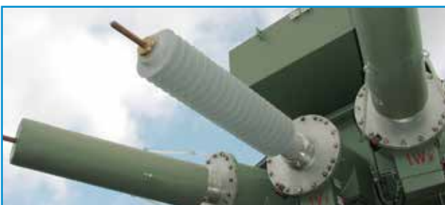
DURESCA® Transformer bushings
