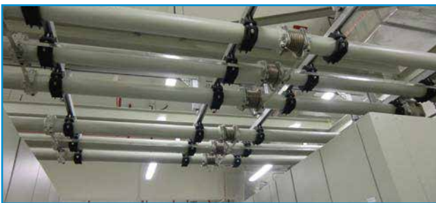
LINK® SF 6 insulatet busbar system
